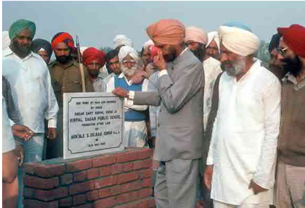
Right: Laying the foundation stone for the future Kirpal Sagar Academy, 1983 Below: Kirpal Sagar Academy, 2007
