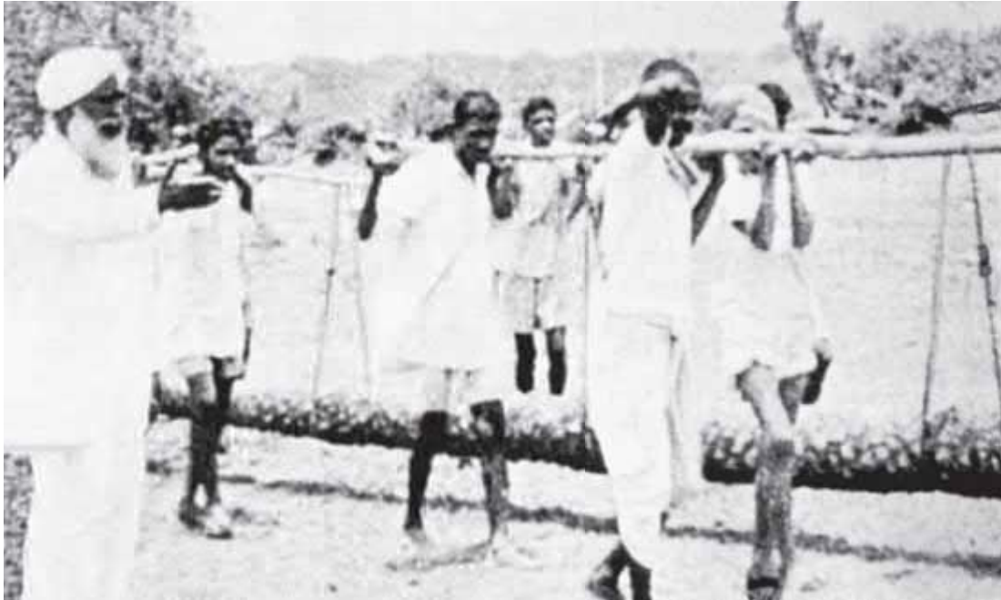
Constructing the Sawan Ashram
