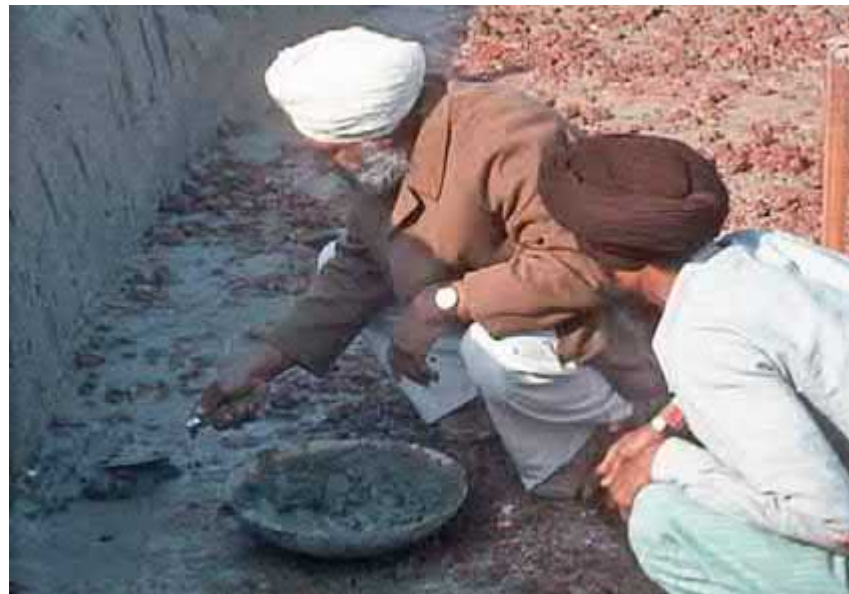
Left: Sarovar at the beginning of the construction work, February 1982 Above: Dr. Harbhajan Singh with the first basket of the bricks, starting the construction work Below: Dr. Harbhajan Singh starting the work of the surrounding wall in the Sarovar on 25 February, 1983
