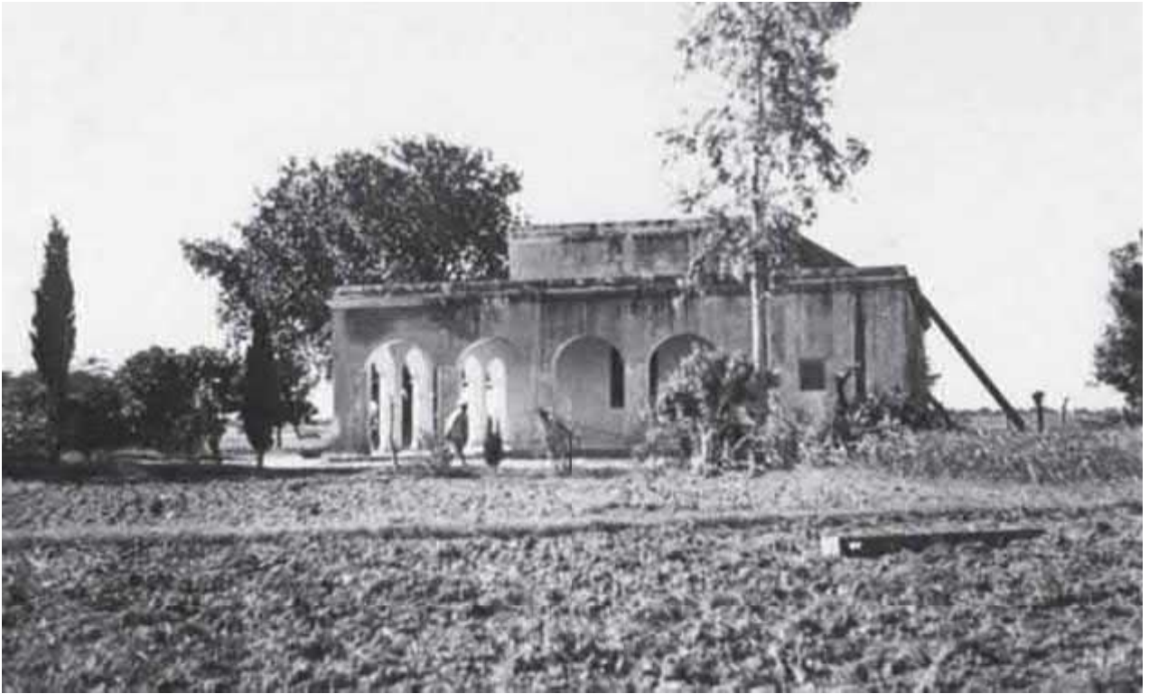
Kothi house near the Beas railway station
